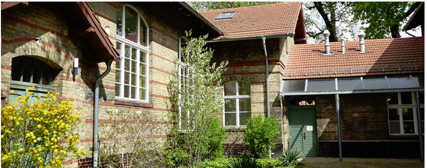
Yard of the BCCN Berlin building
