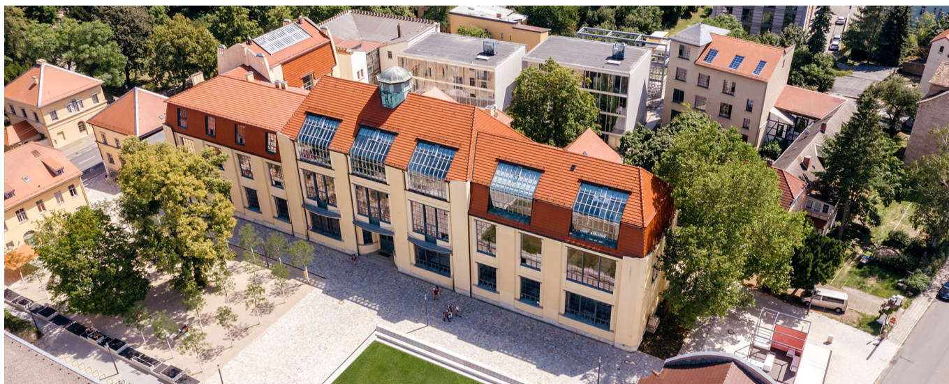
Main building of the Bauhaus-Universität Weimar (UNESCO World Heritage Site)
