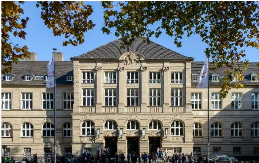
Main building, Südstadt Campus, TH Köln
