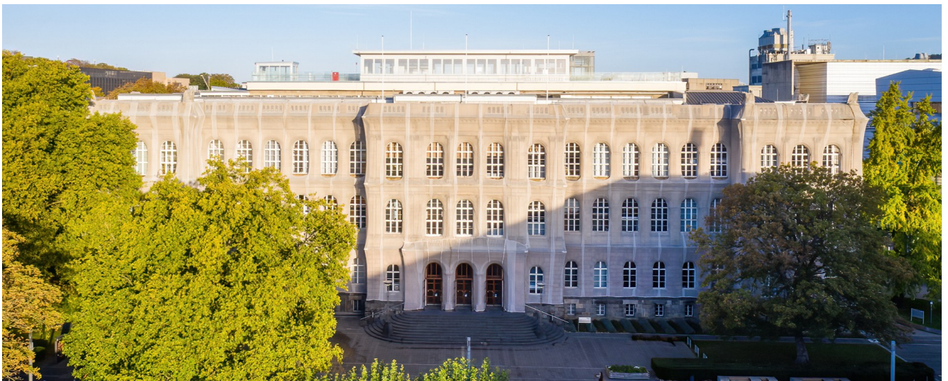
Main building RWTH Aachen University
