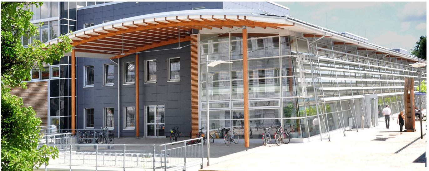
S-Building TH Rosenheim
