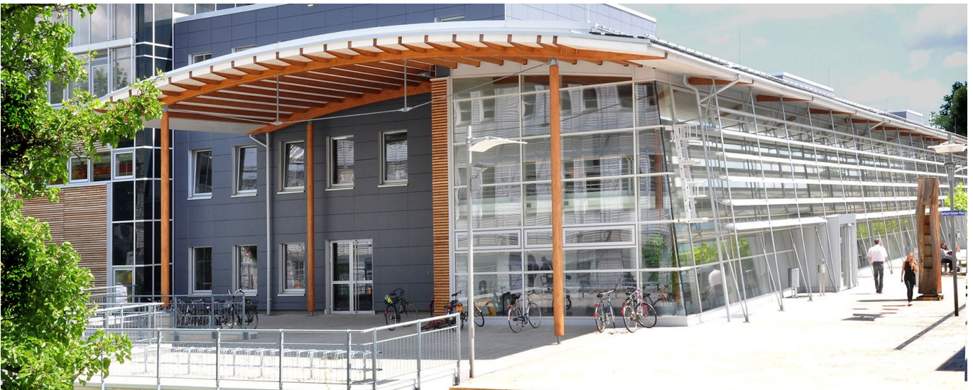
S-Building TH Rosenheim
