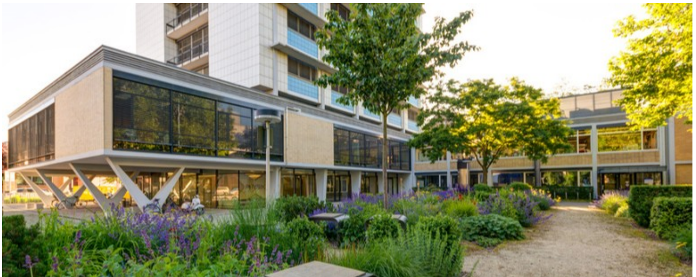
Physics main building
