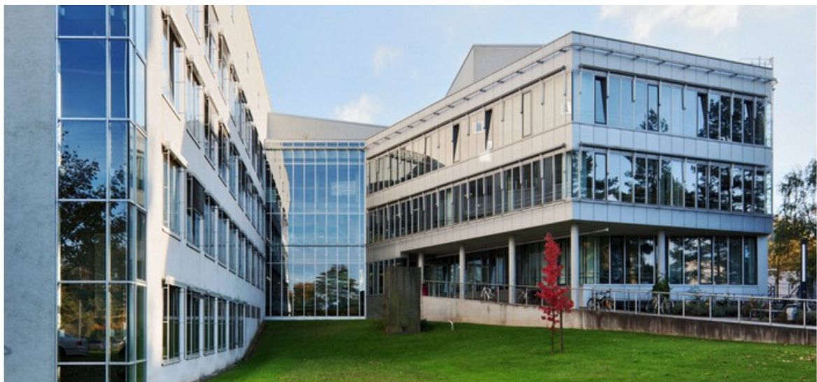
Materials Science main building
