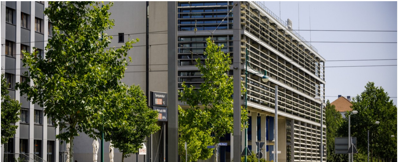
Building of the Faculty of Electrical Engineering and Information Technology
