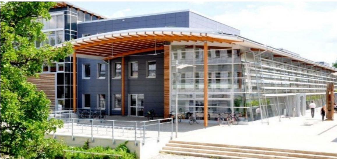
S-Building (Rosenheim Technical University of Applied Sciences)
