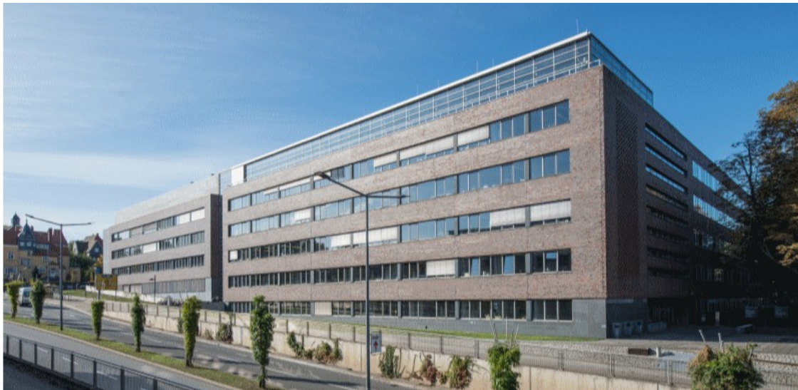
TU Dresden Chemistry Building
