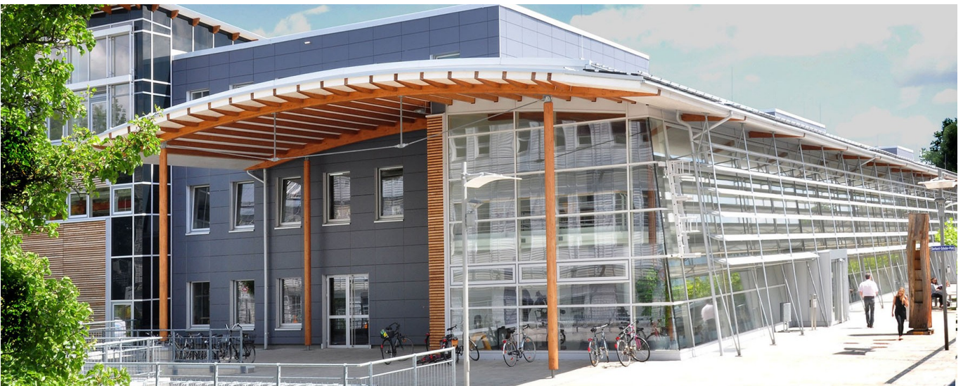
S-Building (Rosenheim Technical University of Applied Sciences)
