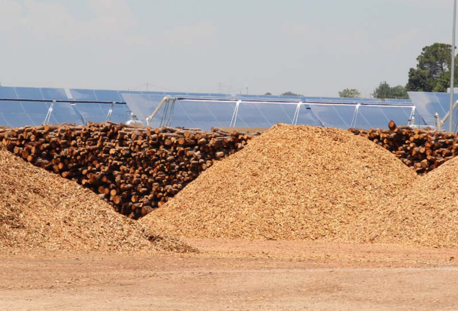
Cogeneration power plant Borges Termossolar, which uses biomass and solar energy as fuels to produce electricity
